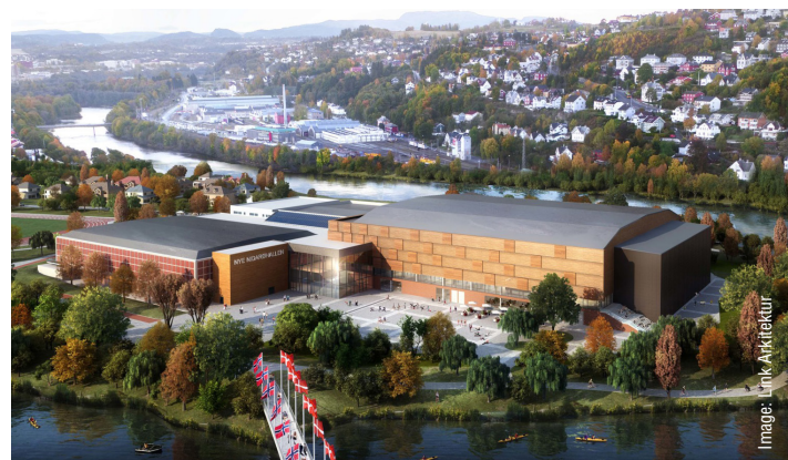
Trondheim is getting a new multi-functional sports centre called Nye Nidarøhallen. Bravida subsidiary Oras is planning and installing all heating and plumbing, HVAC and building automation solutions for the project. The new facility will accommodate everything from local amateur sport and various trade fairs to concerts with 12,000 visitors. The venue is estimated to be completed by autumn 2019.
