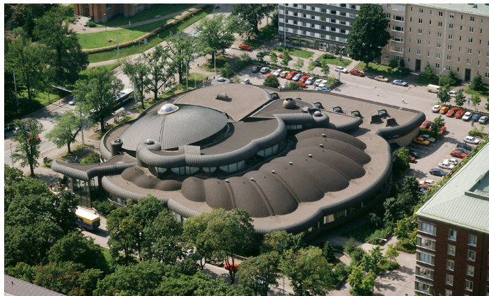
Tampere City Library Metso was constructed in 1986. The building is a valued cultural site that is known for its architecture. The library was recently renovated and Bravida was contracted to carry out all the electrical installations.
