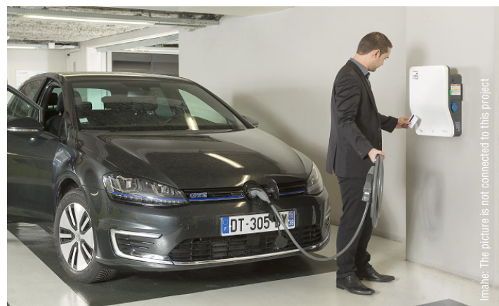
Some 90 charging points for electric cars are being fitted at Telenor's headquarters in Forneby, Oslo. The solution has been planned and designed by Bravida and the installation is expected to be completed by the end of September. Fortum is supplying the power for the facility and is also the customer for Bravida's services.
