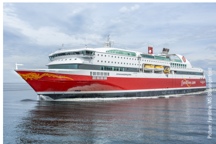
Shipping company Fjordline operates on the Denmark-Norway route. The company has had a service agreement with Bravida for the past six years. The agreement includes all ventilation onboard its vessels, including cleaning and the installation of UV lighting. There are usually 4–5 Bravida technicians onboard when service work is carried out. The vessel shown in the image, MS Stavangerfjord, is one of the ferries serviced by Bravida.
